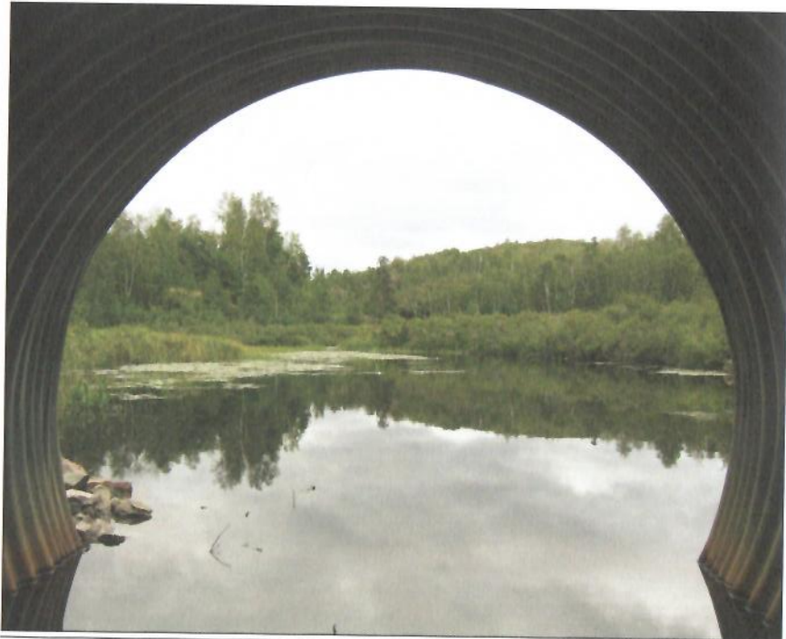
TUNNEL VISION - Fiona Taylor
